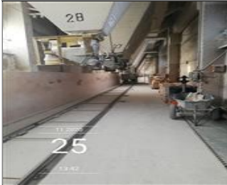
Photo of the inside of the main production hall IMG_20201125_134250.jpg
