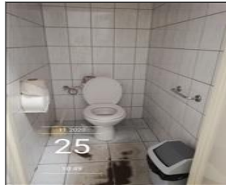
Photo of the sanitary facilities IMG_20201125_104955.jpg
