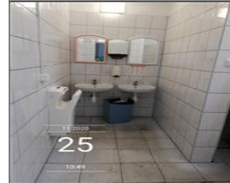
Photo of the sanitary facilities IMG_20201125_104947.jpg
