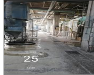
Photo of the inside of the main production hall IMG_20201125_133902.jpg
